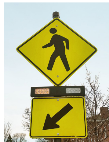
Rectangular Rapid Flashing Beacon
